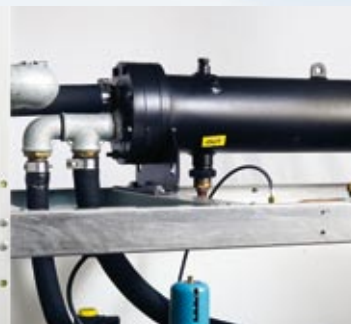
Shell & tube condenser
